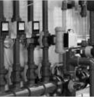
Installation of acid-proof piping, e.g. in the chemical industry.
