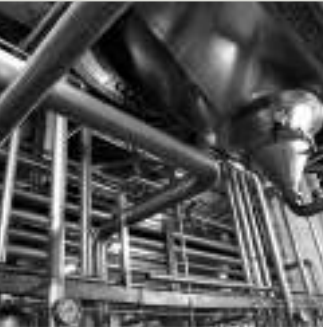
Construction of chemical plants and refrigeration systems.
