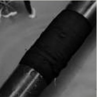
Temporary repair of pipe systems.
