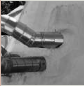
Mortar bulkhead around a metal pipe passage.
