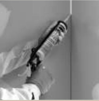
For sealing structural joints, e.g. wall connections.
