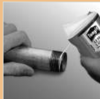
Sealing of connection threads in HVAC engineering.
