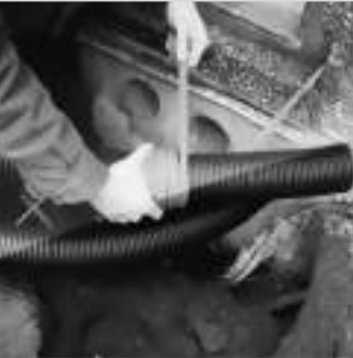
Wrap the M4082 sealing hose around the pipe, ...
