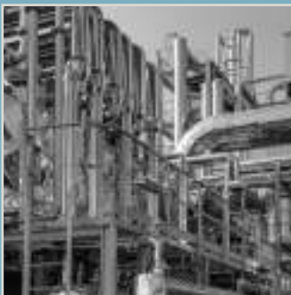
Construction of chemical and metal processing plants.
