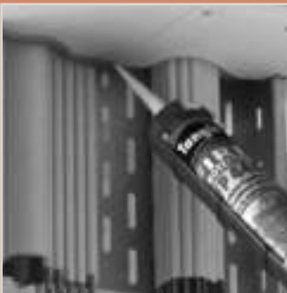
FP440 fills joints between the panels used for cladding the penetration of a ceiling.
