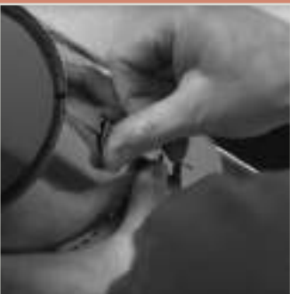
Insertion collar for tool-free installation from one side: align – insert – finished!
